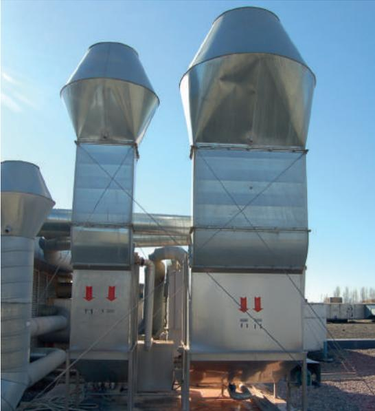
Wet filters are used for the dusts which cannot be filtered dry by cartridge or bag filters due to the physical and chemical properties. These filters are suitable for explosive atmospheres also.
