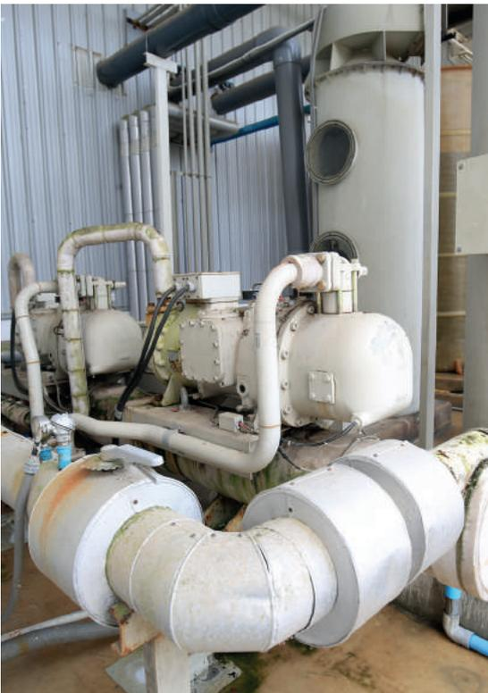
Gas Scrubber Systems are the most common exhaust treatment systems used for the removal of combustion gases, process waste gases, vapors and other pollutants that are generated during the activities of various industrial productions. For the chemical, metallurgy, iron and steel, food, textile, paint, cosmetic, chemical storage, artificial leather, precious metals (gold, silver), foundry, thermal processing, surface finishing facilities we can supply tailor made solutions
