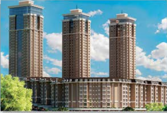
İSTANBUL GREY YAPI / TRENDİST ATAŞEHİR 22 PCS. MULTIBLOC STEEL BOILER
