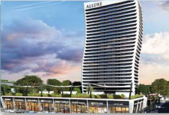
İSTANBUL DORUK İNŞAAT / ALLURE TOWER 5 PCS. MAGNUS
