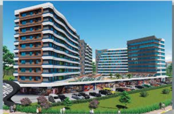
İSTANBUL AYDINOĞLU İNŞAAT / KURTKÖY AYPÖRT RESIDENCE 40 PCS. LECTUS 115
