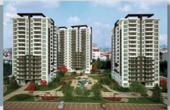
ANKARA ASM İNŞAAT / PLATİN KONUTLARI 2 PCS. STEEL BOILER / 1690 MTUL PANEL RADIATORS
