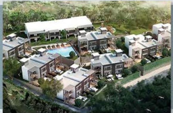
ÇANAKKALE BEGONVILLE VADI EVLERİ 21 PCS. HEAT PUMP
