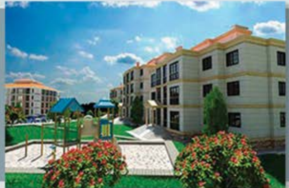
AFYON TOKİ KONUTLARI 23 PCS. MULTIBLOC BOILER
