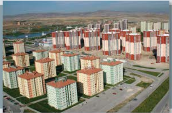
DİYARBAKIR DİBAY İNŞAAT / TOKİ KONUTLARI 234 PCS. DAB FREQUENCY CONTROLLED PUMP 121 PCS. DAB DRAINAGE PUMP
